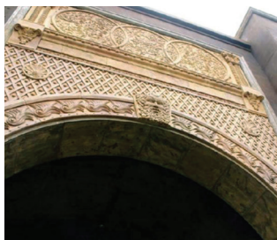
ARCHITECTURAL REPRODUCTION & RESTORATION
